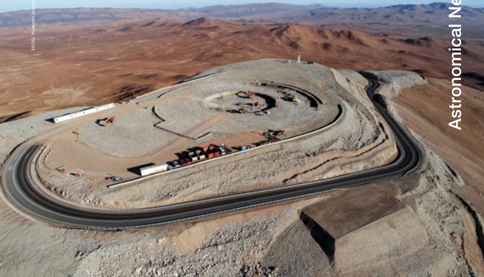
Upper image: Construction proceeding at the site of ESO's ELT.
